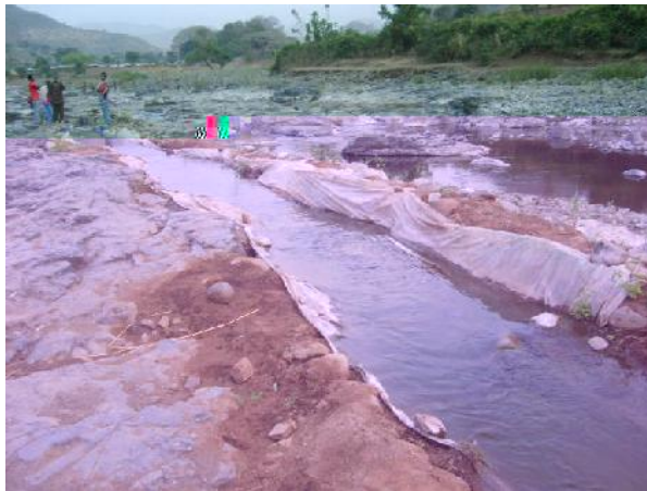
Figure 5. Diversion structure and primary canal at Zarima
