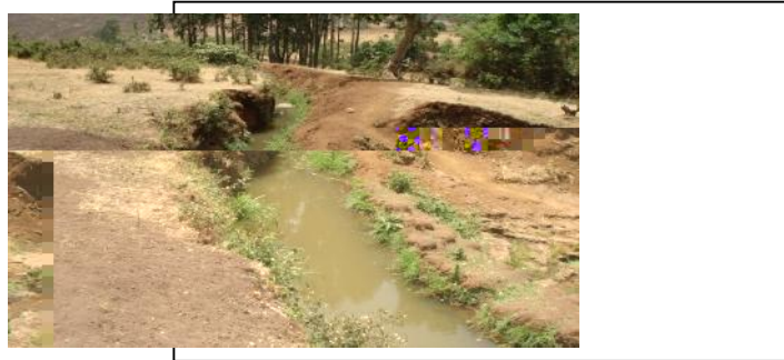
Figure 14. Unstable ditches
